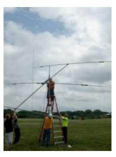
balloon and kite experiments. Unfortunately one of the ropes planned for the wire antennas at the top of the tower pulled off; however, ingenuity saved the day and a system using the steel guy cables from the tower was devised as a clever way to hoist the wire up. Consequently the 80 and 40 meter vee's were in place in short order. (My dream of building a 20M delta-vee did not materialize due to time constraints).
