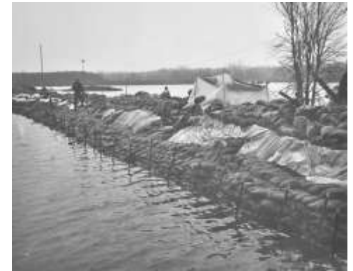
More than 1.3 million sandbags raised Winona’s dikes against the 1965 flood.
