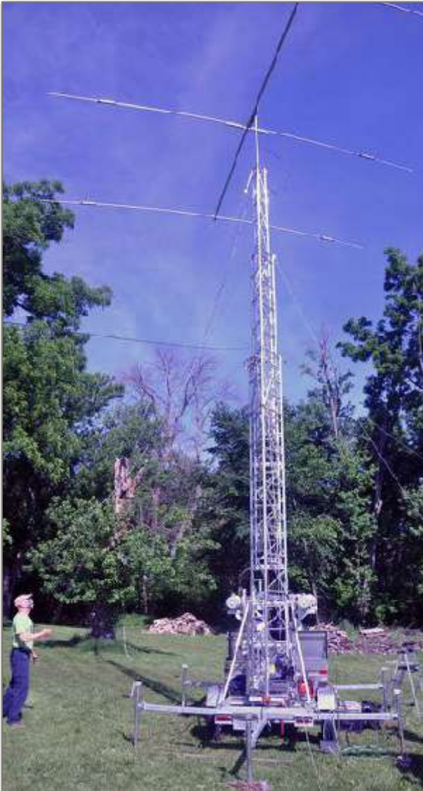
RAISING THE COUNTY MOBILE TOWER BEFORE THE RAINS CAME.
