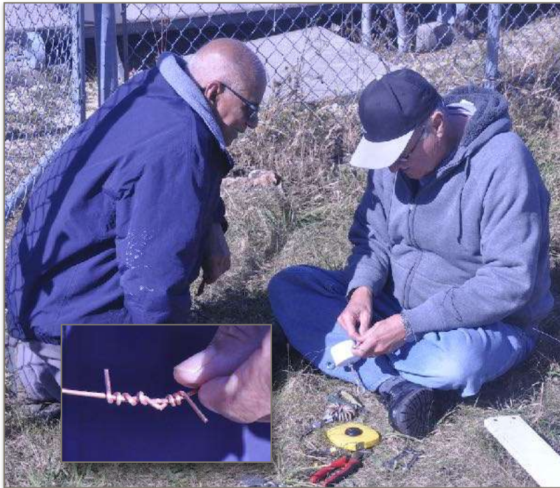
A 160 METER DIPOLE IS PREPARED FOR THE CLUB'S WITOKA HF REMOTE STATION BY SYED FARUQUE, AC0VA, LEFT, AND MIKE FOERSTER, W0IH. THEY CONVERTED THE 250' OF ENDFED ANTENNA WIRE INTO A 160 METER CENTER FED DIPOLE, INVERTED VEE FORMATION.
